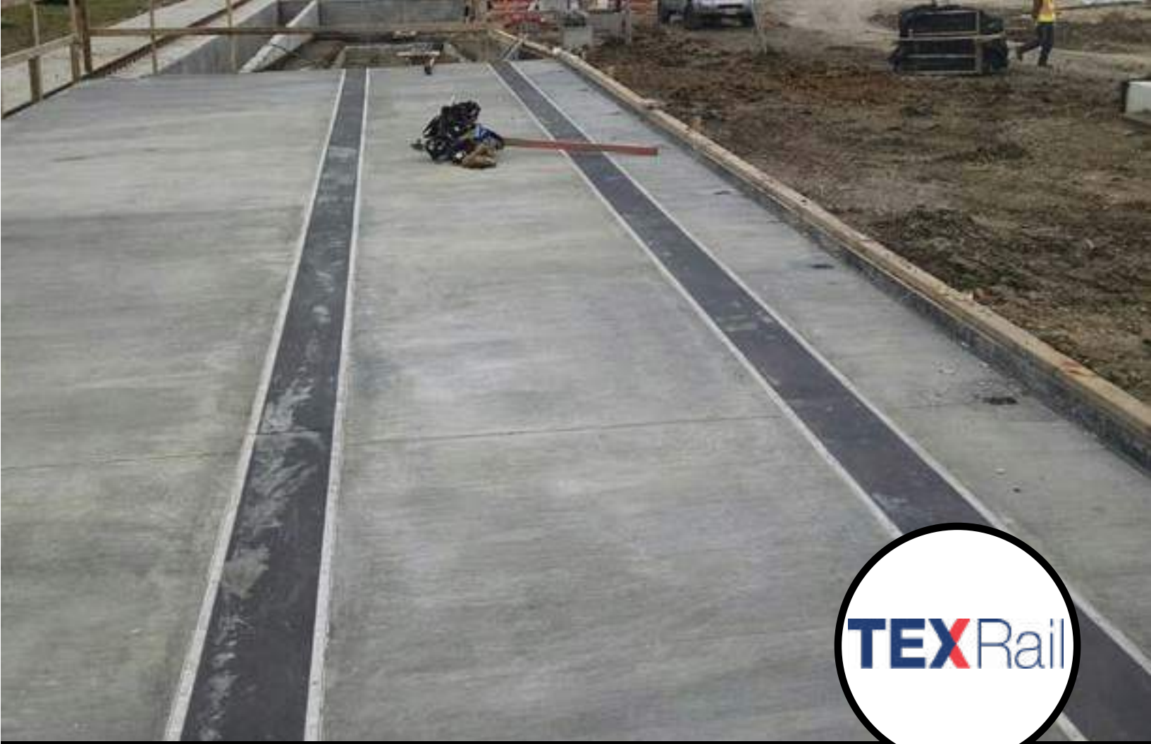
Trench covers with abrasive infill (TSA) installed at TEXRail Stations circa Dallas/Fort Worth, TX
